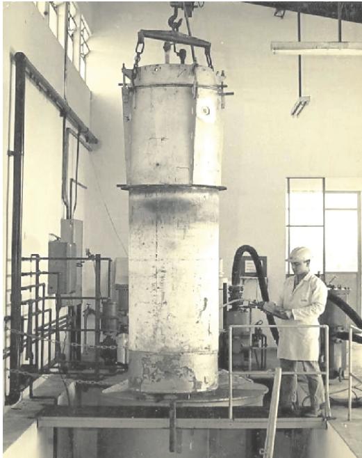
Figure 2: Reactor-retort, equipment developed by CTA for titanium sponge production (Henriques, 2008).
